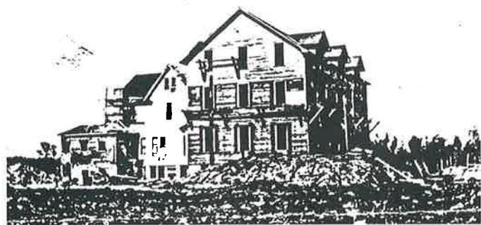
Walderly School Annex
