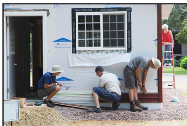
Volunteers finishing the siding on the new Medical Building! Thank YOU!
