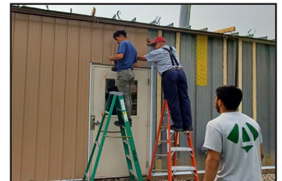
New siding on the Tech Ed. Building
