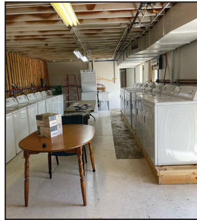
New Laundry Room in Cedar Lodge
