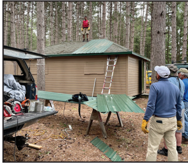
Thank You Volunteers! - New Cabin Roof
