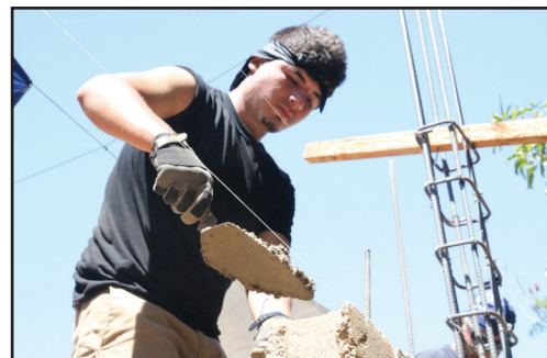
Junior Mikel Arce fills block with cement at the construction site. Students and community members worked together, building the first Seventh-day Adventist church in Marcilla.
