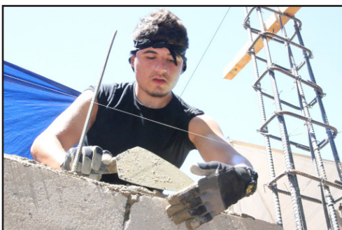
Mickel Arce ('17) helps build a cement block wall on Marcilla church during our 2016 mission project.
