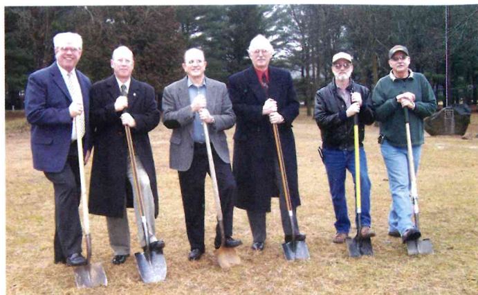
After working for months to secure all appropriate permits, Conference Leaders broke ground for the new Pavilion at Camp Wakonda on November 28. Left to right: James Fox, Roger Driver, Richard Habenicht, Don Corkum, Floyd Brock and Jim Johnson.
