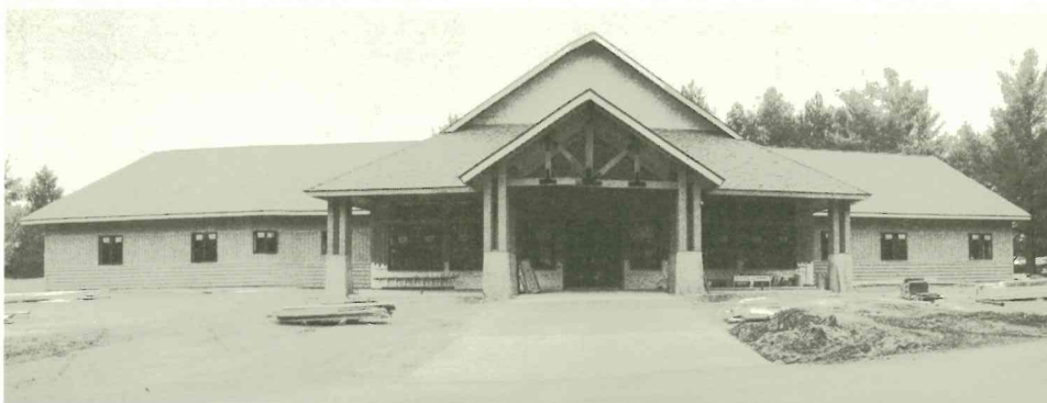
The new Fireside Lodge after 6152 hours of hard work by Maranatha Volunteers and many supportive Wisconsin church members.
